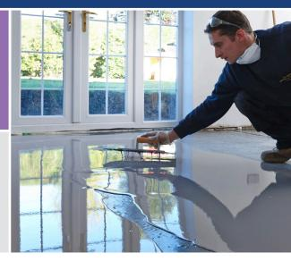
**SETCRETE™ LATEX** is suitable for use over a wide range of absorbent subfloor types including sand/cement screed and concrete. It is also suitable for use over non-absorbent subfloors such as ceramics, granolithic, terrazzo, epoxy and polyurethane resins and quarry tiles, providing they are sound, well adhered and suitably prepared.
